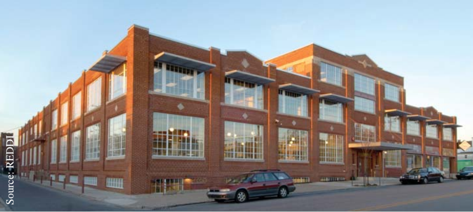
Energy-efficient press building located in Harrisburg, PA
